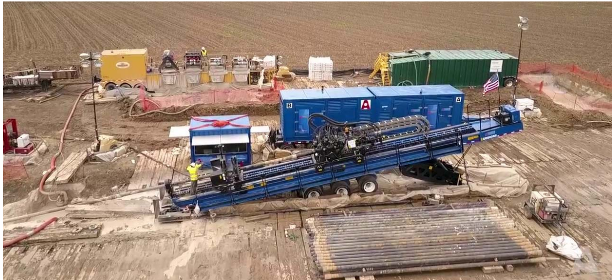
Figure 8: Example of HDD drill rig and supporting equipment.
