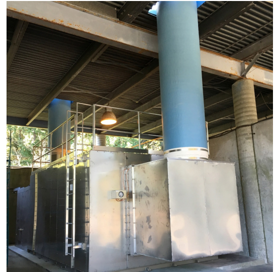
The dual bed activated carbon polisher 'polishes' air by filtering out odour.
