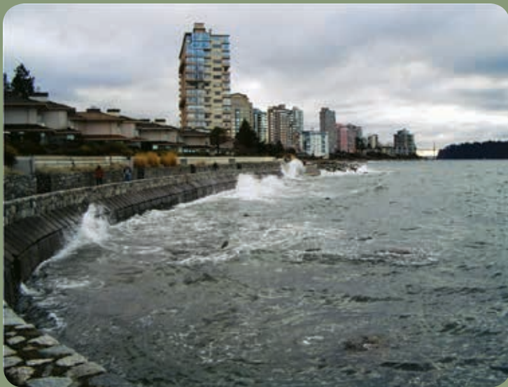
West Vancouver, B.C. Seawall
