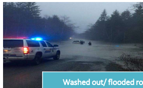
Washed out/ flooded roads
