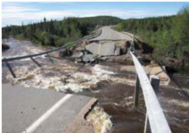
FIGURE 7: Damage to the highway and bridge near Port Rexton, NL due to Hurricane Igor. Photo courtesy of Fire and Emergency Services, Newfoundland and Labrador.
