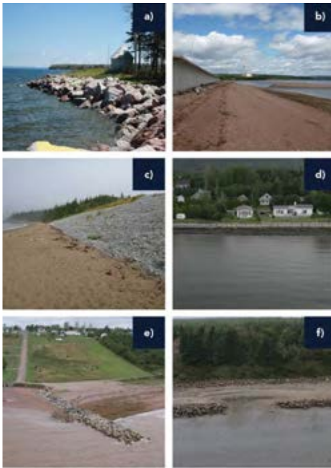
FIGURE 22: Coastal-protection structures commonly used in the East Coast region ( adapted from Jennings et al., 2008 ): a) riprap, Malagawatch ancestral burial grounds, southwestern Bras d'Or Lake, NS (S. O'Carroll, Geo Littoral Consultants); b) seawall, Eel River Bar First Nation, northeastern New Brunswick (D. Bérubé, New Brunswick Department of Energy and Mines); c) revetement, Mispec, southwestern New Brunswick (D. Bérubé, New Brunswick Department of Energy and Mines); d) bulkhead, Maria, Gaspésie, QC (Laboratoire de dynamique et de gestion intégrée des zones côtières—Université du Québec à Rimouski [UQAR]); e) groyne, Paspébiac, Gaspésie, QC (Laboratoire de dynamique et de gestion intégrée des zones côtières—UQAR); and f) breakwater, Pointe-Lebel, north shore of the St. Lawrence estuary, QC (Laboratoire de dynamique et de gestion intégrée des zones côtières—UQAR).
