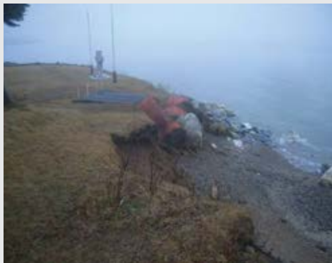
FIGURE 15: Malagawatch Cemetery, NS, where buried human remains eroded into the sea following several storm events. Initial protection of the site involved the use of stone armouring (as seen below the cross). Subsequent storms and erosion led to temporary protection of burials using anchored hay bales and a permeable membrane (centre of photo). Planning for more permanent protection is ongoing. Photo courtesy of Heather MacLeod-Leslie.
