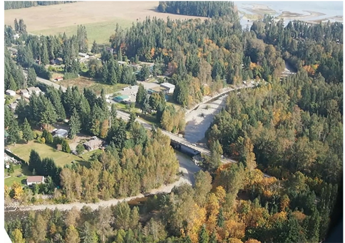
Figure 20: Oyster River Bridge
