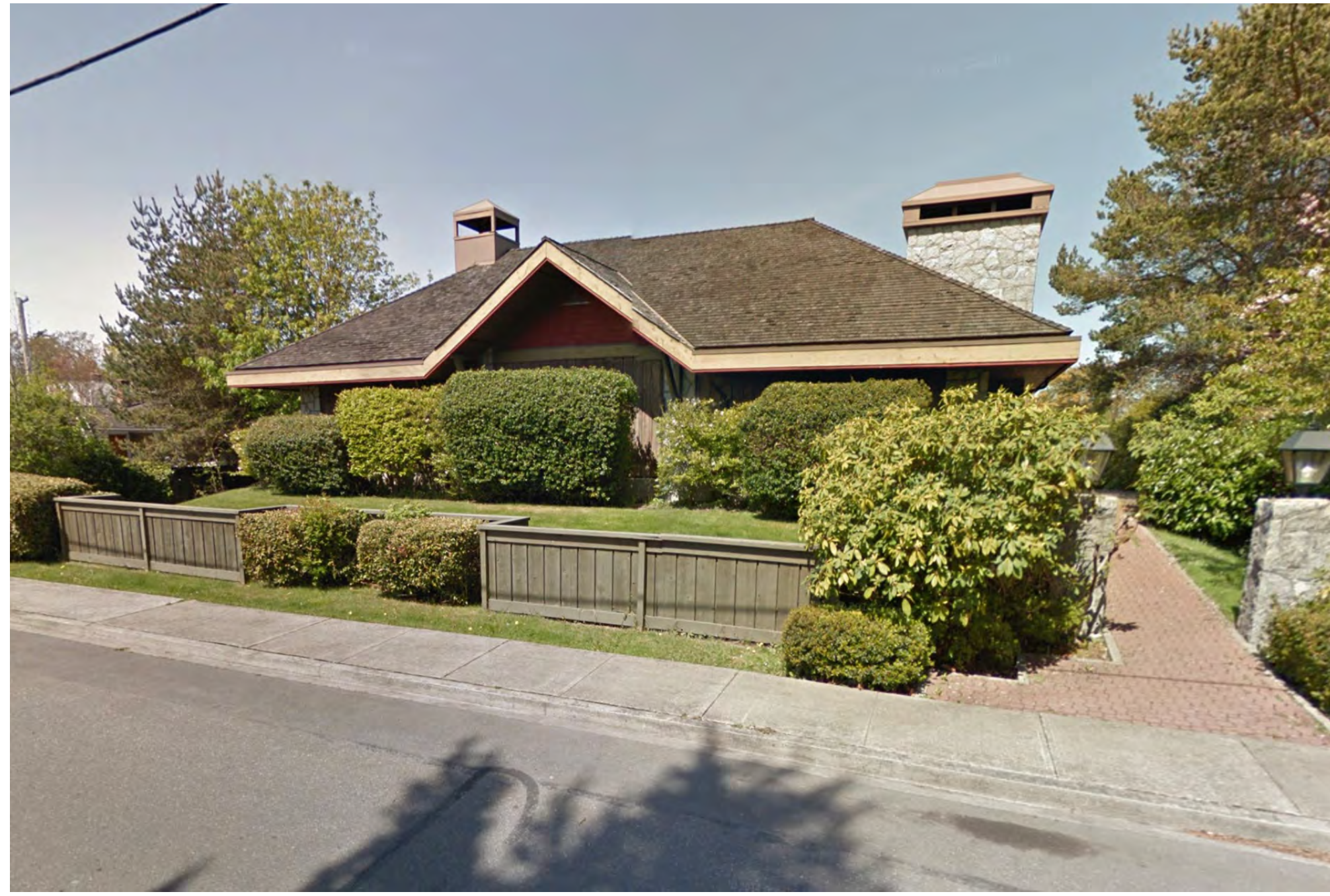
CURRIE ROAD PUMP STATION - OAK BAY BC
