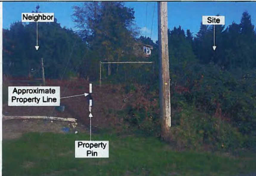
Photo 4: Close-up view of the existing grade change at the north property line with inferred fill on the upslope neighbour's property.
