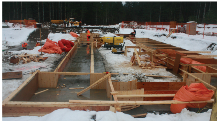
Laying the foundation at the new Water Treatment Plant site.
