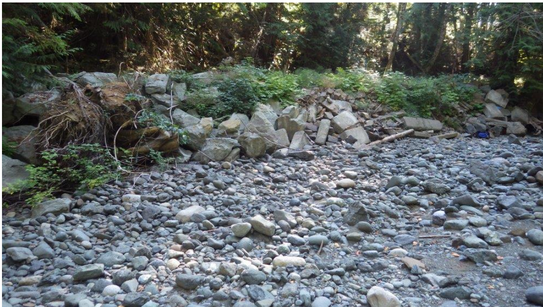
Figure 48. Bank armouring, August 24, 2018.
