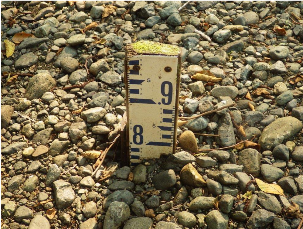
Figure 21. Buried staff gauge (installed ~ 2001) behind log jam demonstrates recent aggradation, August 22, 2018.
