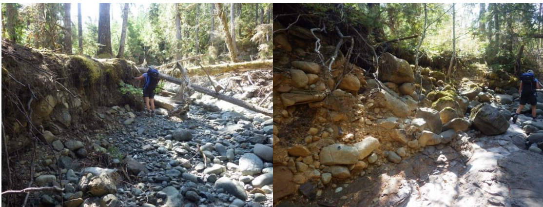
Figure 51. Eroding bank; clear-cut close to stream bank, August 24, 2018.
