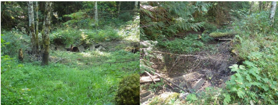
Figure 59. Seepage from Allen Lake middle dam tributary, August 24, 2018.
