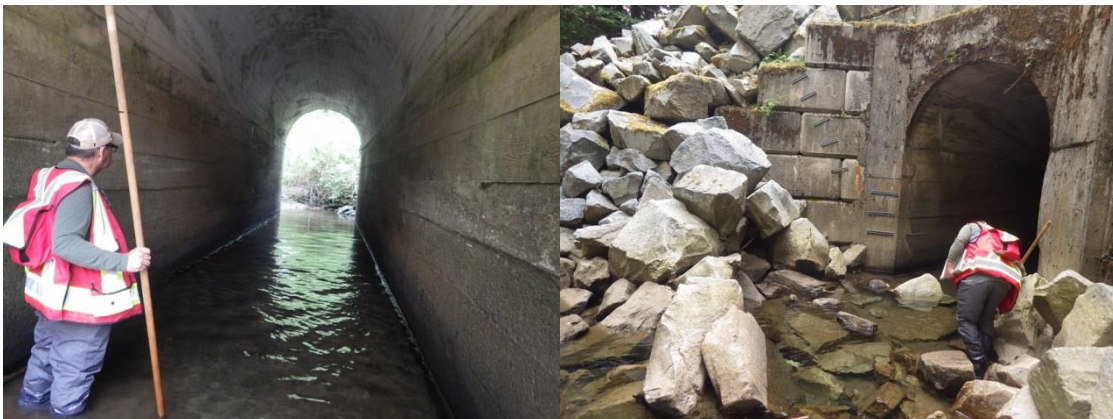
Figure 12. Culvert under Comox Lake Road, August 22, 2018.
