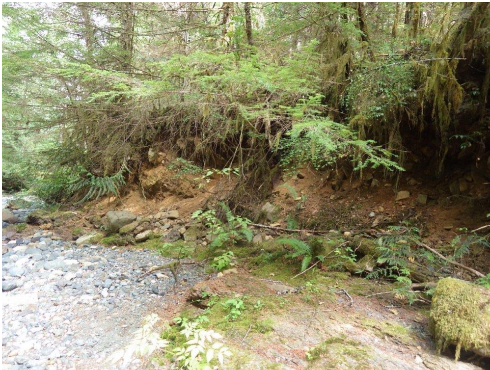
Figure 37. Eroding bank (3m high x 20m wide), August 23, 2018.
