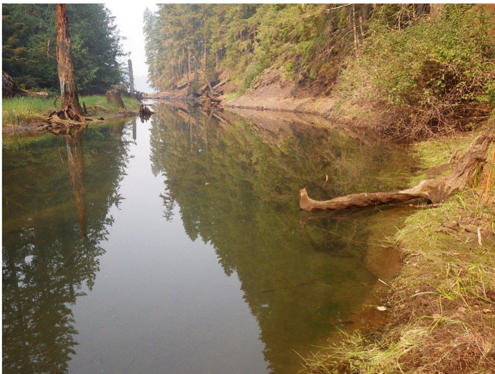
Figure 4. Eroding banks on old coal slag piles, August 21, 2018.
