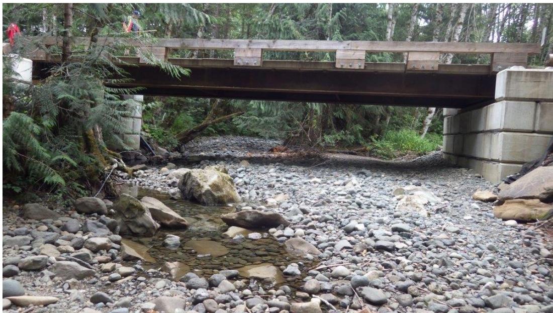
Figure 42. Davis Creek Main bridge, August 23, 2018.
