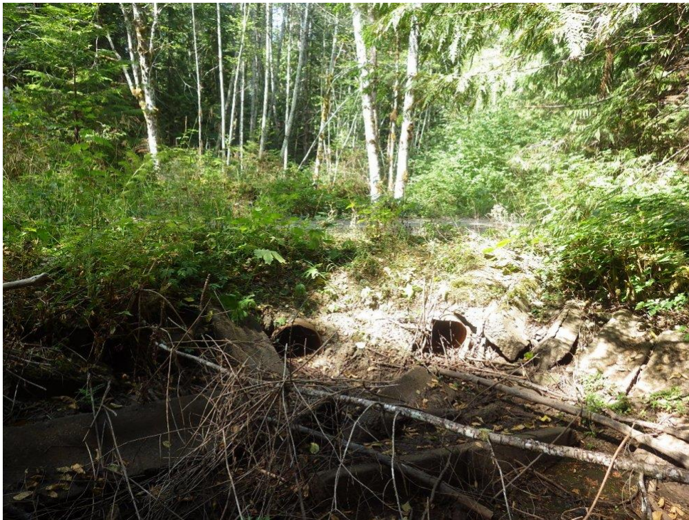
Figure 53. Allen Lake west tributary outlet beneath access road, August 24, 2018.
