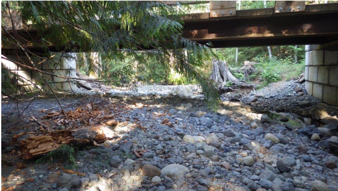
Figure 43. Davis Creek main bridge, August 24, 2018.
