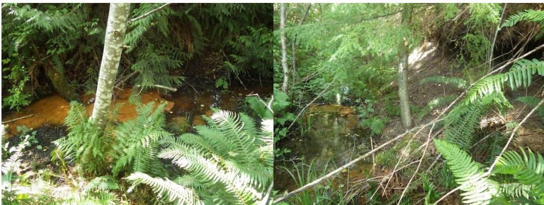
Figure 60. Seepage flow from East dam; iron algae blooms August 24, 2018.
