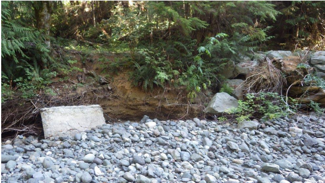
Figure 47. Eroding bank (left) and bank armouring with pavement (right), August 24, 2018.
