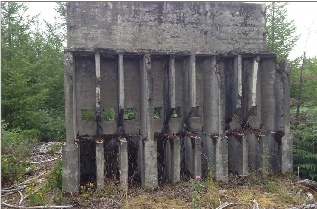
Photo 15: Historic substation building at Scott's Slope.
