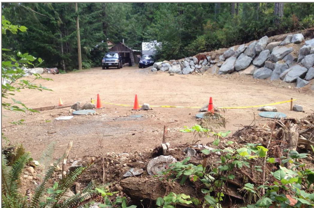
Photo 4: Example of a septic distribution field on south portion of the Property.
