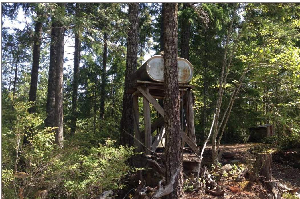
Photo 11: Heating oil style tank used for potable water for a cabin on the north portion of the Property.
