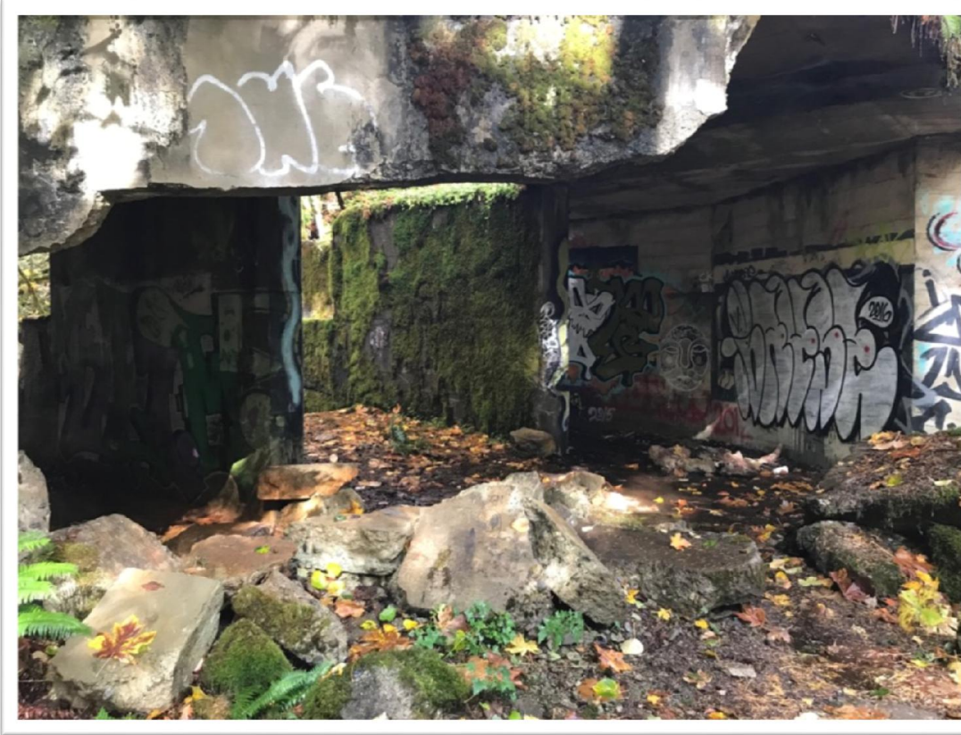
Figure 3 Concrete Ruins of No.4 Mine Fan House
