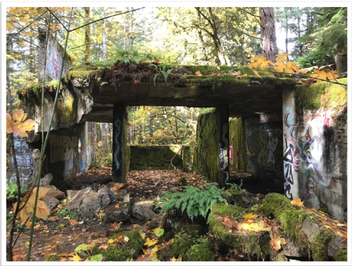
Figure 1 View of #4 Mine Fan House along the rail to trail path to Coal Beach
