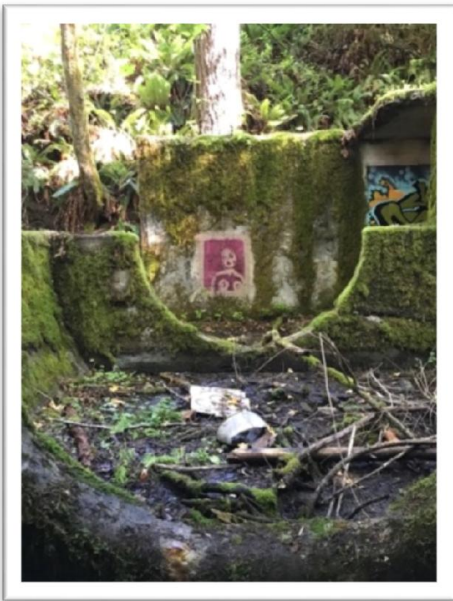
Figure 2 Concrete Ruin of No.4 Mine Fan House showing curved concrete walls
