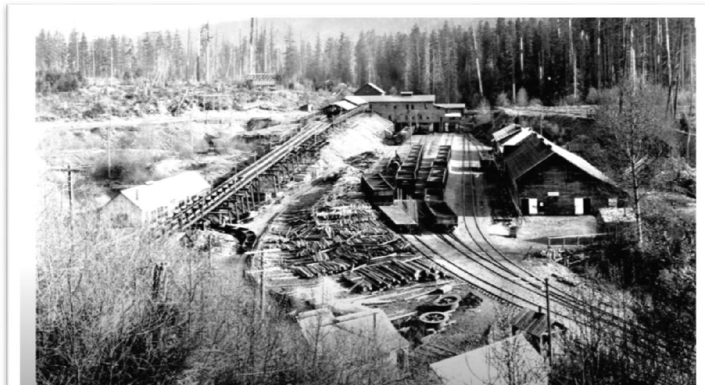
Figure 13 General View of No. 4 Mine. C164-040, Cumberland Museum and Archives.
