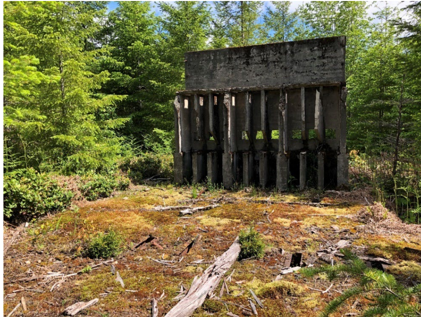
Figure 3. HBF3: cement building on cement platform near Scott's Slope mine entrance, May 22, 2020.
