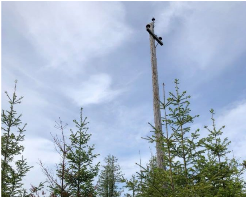
Figure 8. HBS8: Transmission line pole at east edge of the property, May 19, 2020.
