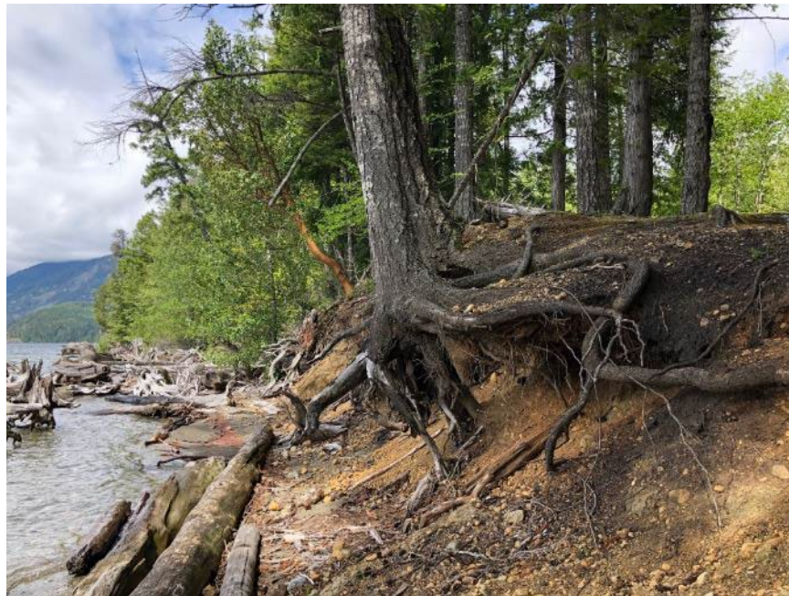
Figure 39. Coal slag erosion along shoreline at Scott's Slope, May 22, 2020.
