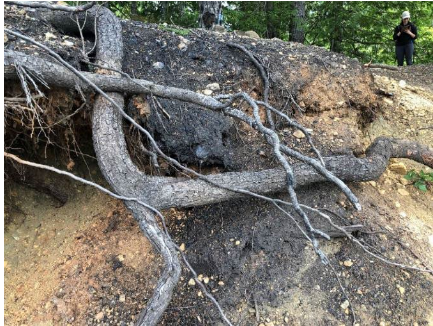
Figure 5. HBF5: Small amounts of coal slag visible in APEC area on north shoreline of property, May 22, 2020.
