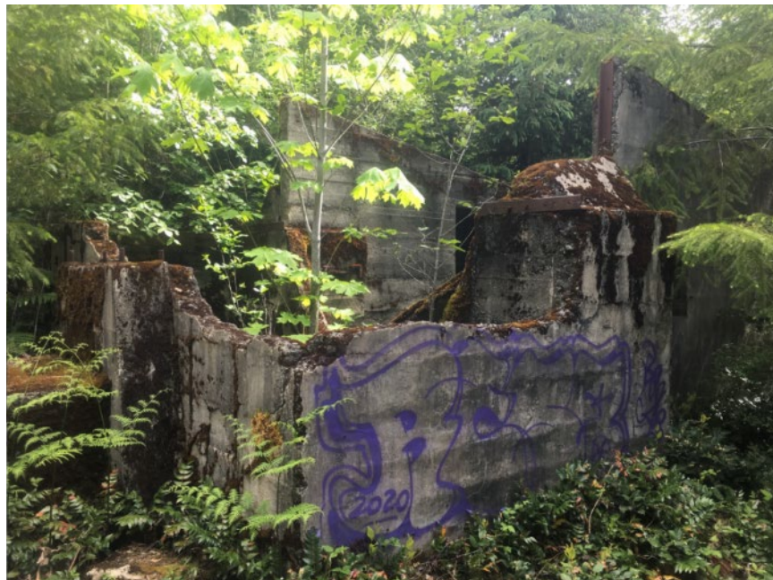
Figure 2. HBF2: Building along access road near Scott's Slope mine entrance, May 22, 2020.
