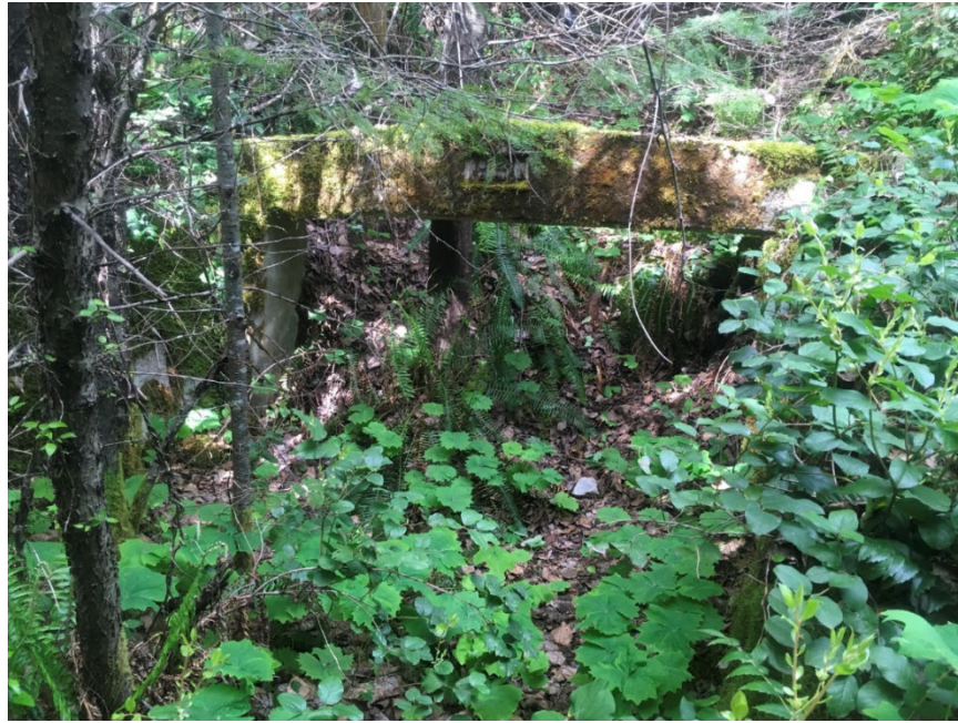
Figure 1. HBF1: Scott's Slope mine entrance with collapsed tunnel behind, May 22, 2020.
