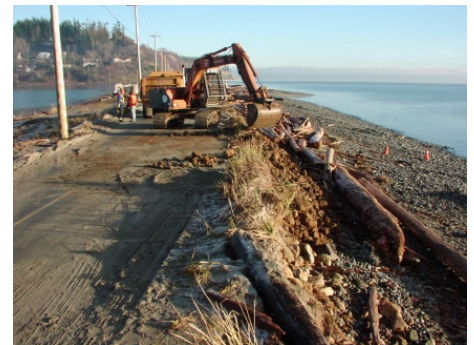
Ministry of Transportation contractor repairing erosion along Hawkins Road. Goose Spit Park is located on both sides of Hawkins Road.
