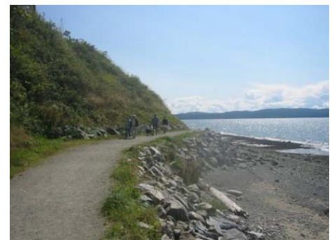
A shoreline trail recently constructed in Powell River in an exposed ocean environment.
