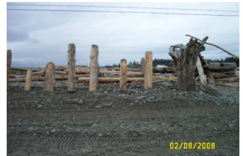
Newly installed log structures. The line of widely spaced logs will be further reviewed for their effectiveness and potentially be removed in favour of other techniques and locations.
