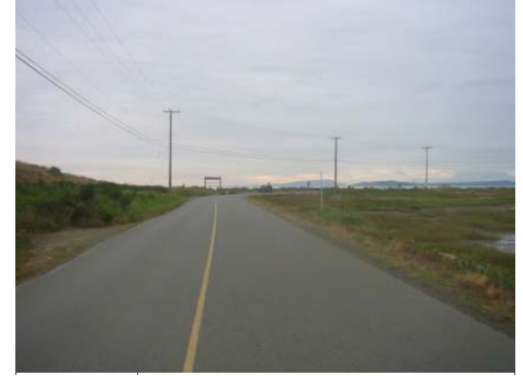
Hawkins Road just before Park entry. A separated walking route could potentially be constructed potentially reducing pressure from private automobiles.
