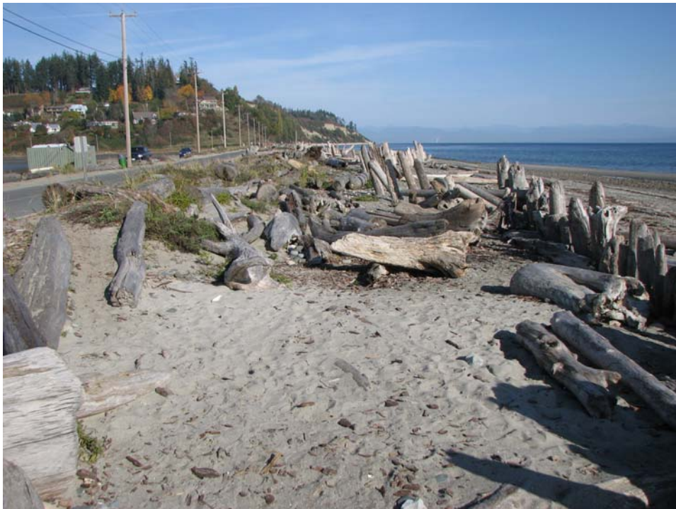
Photo 2: Viewing north east Type 2 log protection
