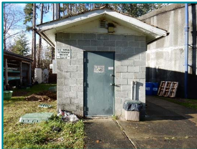
Figure 1: Royston Chlorination Station.
