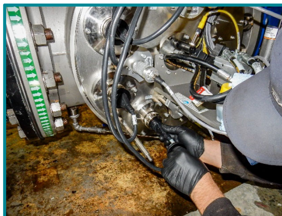
Figure No.2: Installation of UV Equipment
