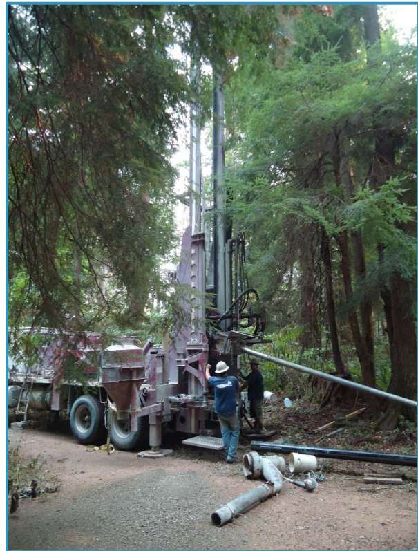
Figure No.8: Drilling of Test Well
